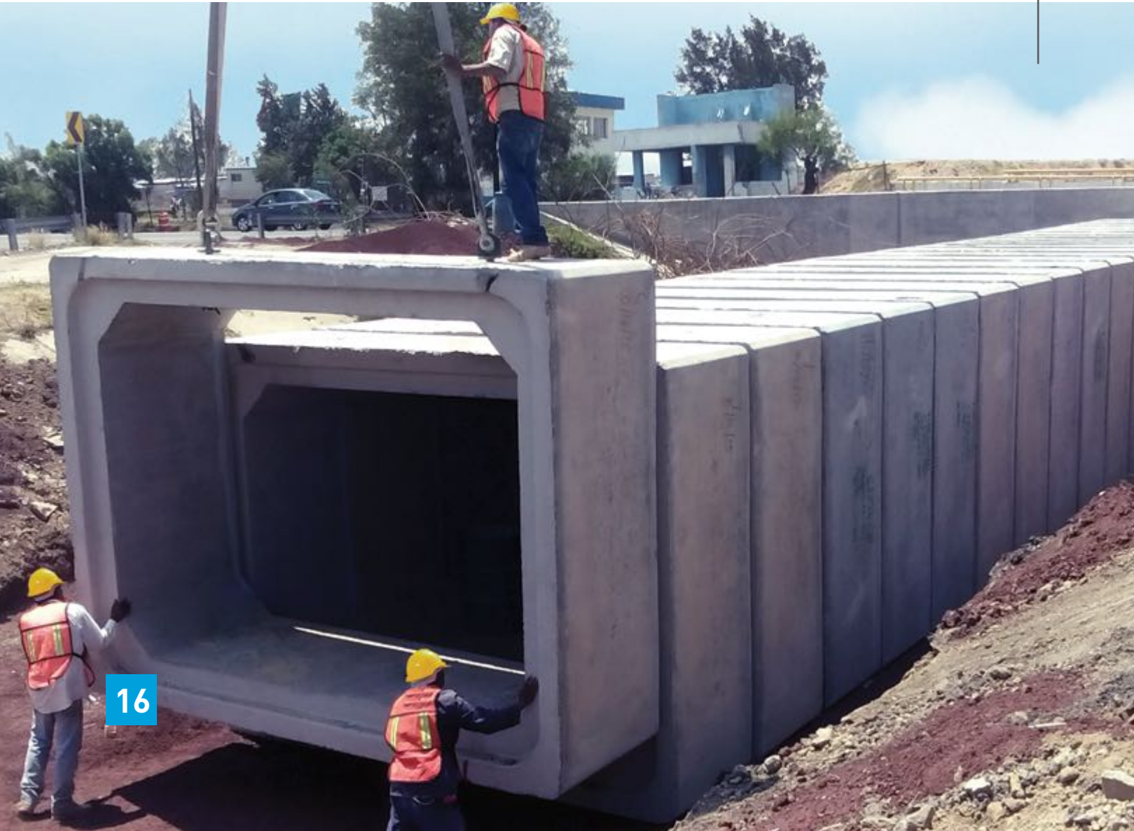
CONSTRUCTION OF CROSSING FOR PEÑON TEXCOCO HIGWAY WITH PREFABRICATED BOX OF 2.11 M, TEXCOCO, STATE OF MEXICO
