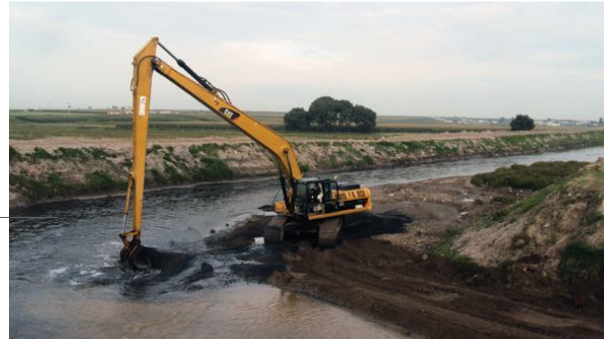
DREDGING OF LERMA RIVER, METEPEC, STATE OF MEXICO
